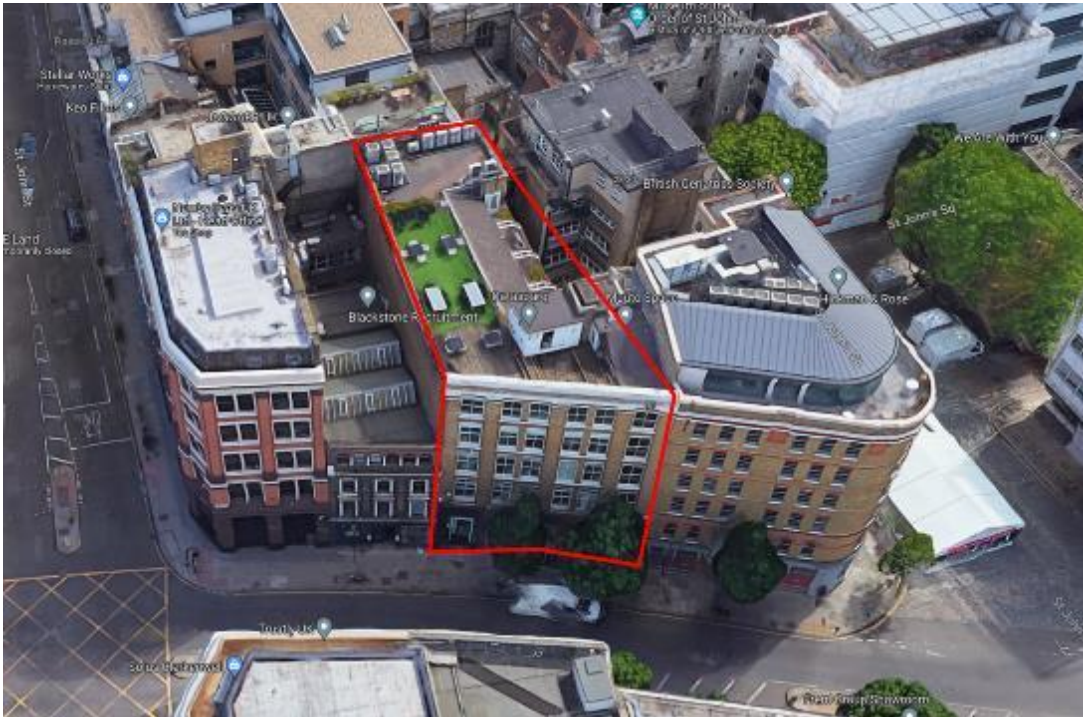
Image 5 - Aerial View of Site in Context
