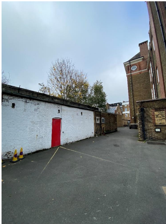
Image 4: View of outbuildings to be demolished
