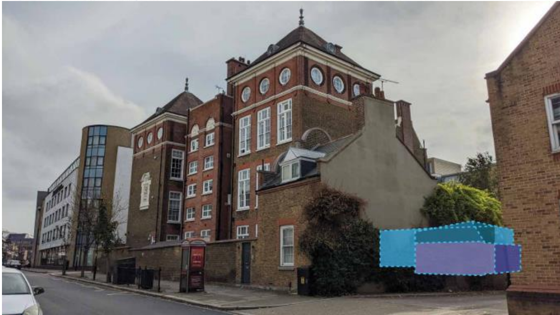
Image 11 and 12: Wireline views of studio from street level
